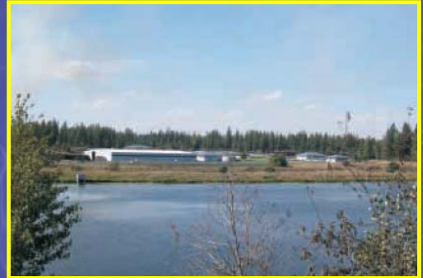
A view of the Cheney wastewater treatment and biosolids reclamation facility from the constructed treatment wetlands
